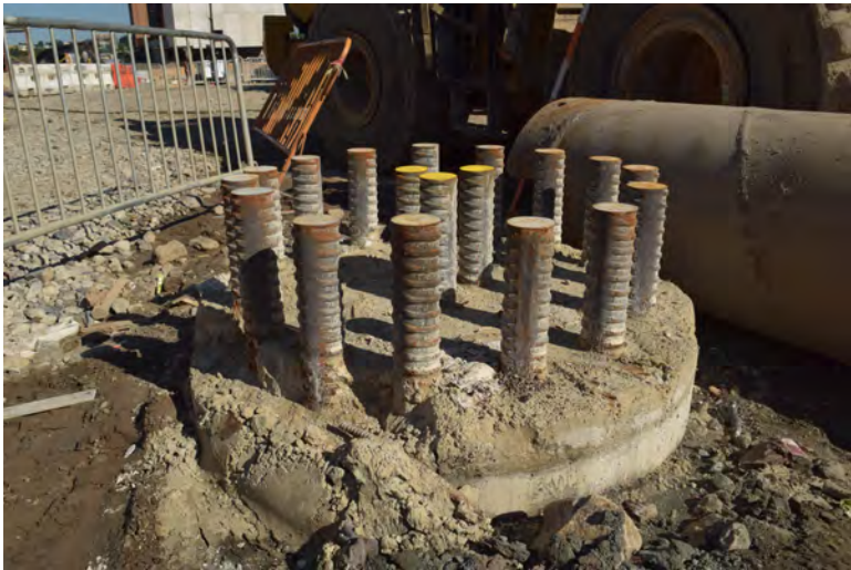
Above: (Left) Caisson cage installed and coupled on site. Kimmel Pavillion, NY, NY (Right) Engineered Drawing Courtesy of FNA Associates Inc.
